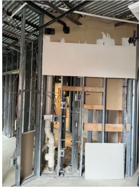
What will be the bathroom.
